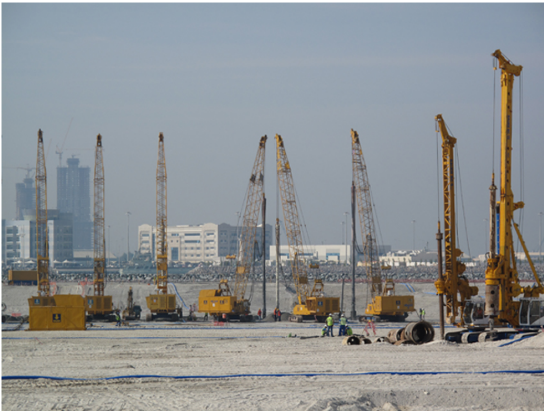
Cranes align on the construction site of the Louvre Museum, Abu Dhabi. The museum, among other construction sites in Saadiyat Island like the Guggenheim Museum, has been criticized for using precarious immigrant labor.
