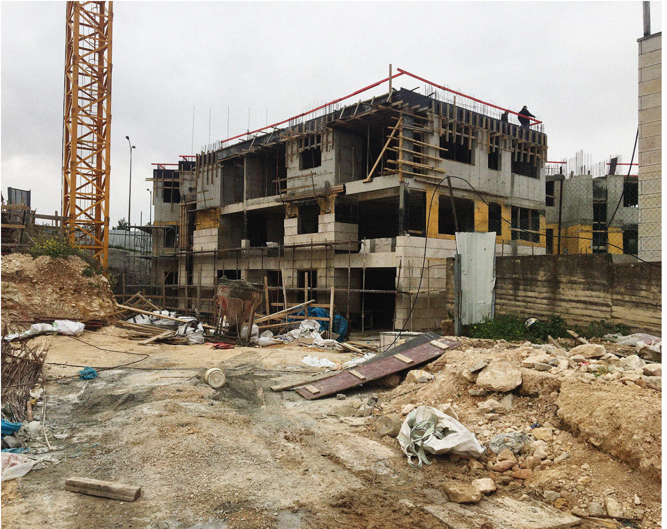
A construction site in Shu'fat. Courtesy of the author.
