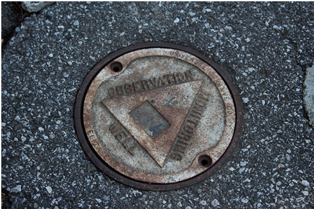
Groundwater monitoring well, Cupertino.
