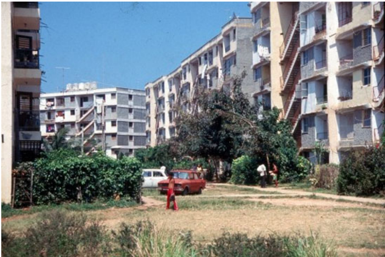
These apartment buildings were built by the Microbrigade systems, Alamar, 1970s. Photo: Roberto Segre
