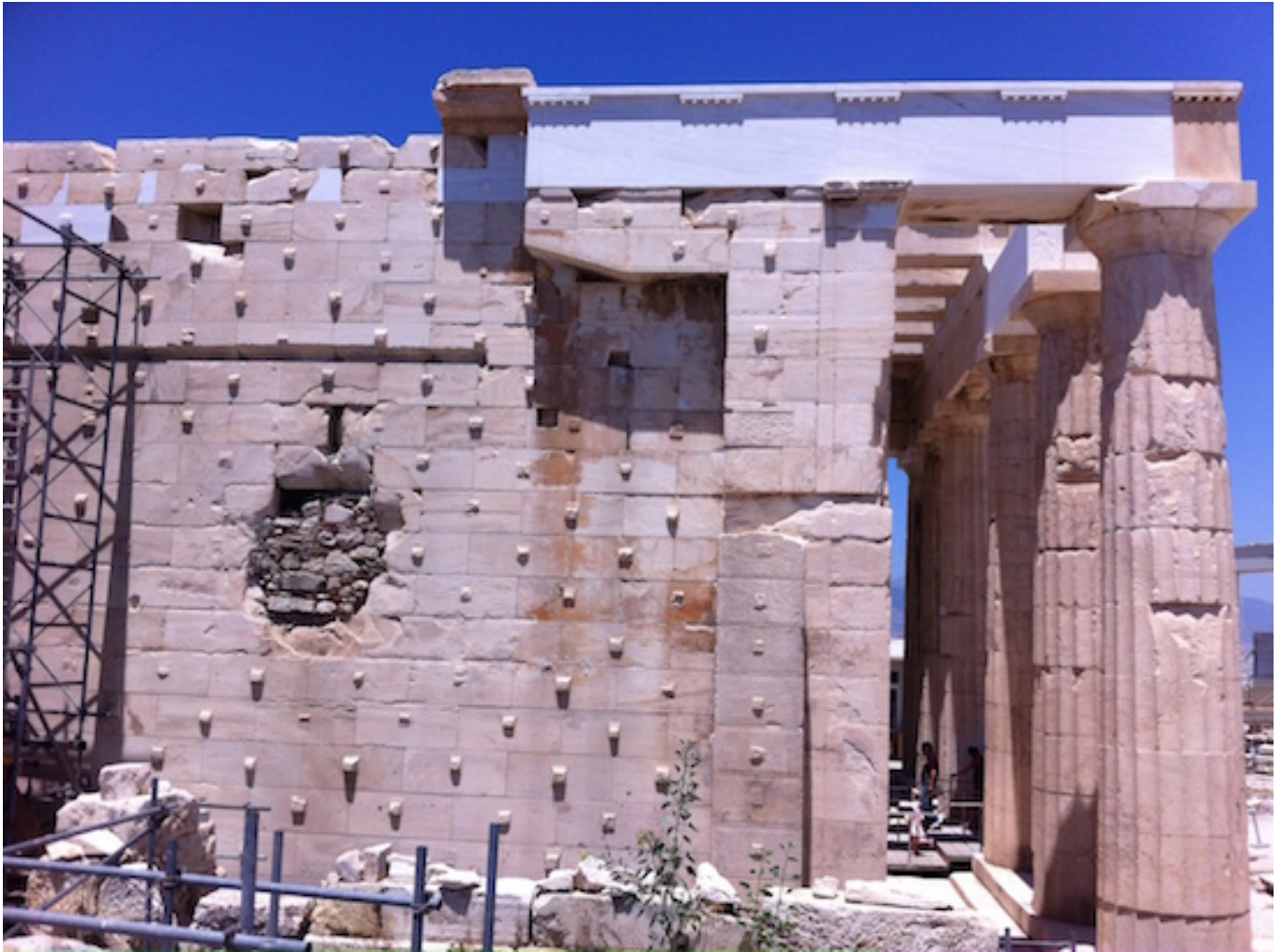
The apergon of the Propylaea at the Acropolis protected the stones during transport and construction and was meant to be struck from the work in a future that has yet to come. Photo: Jorge Otero-Pailos
