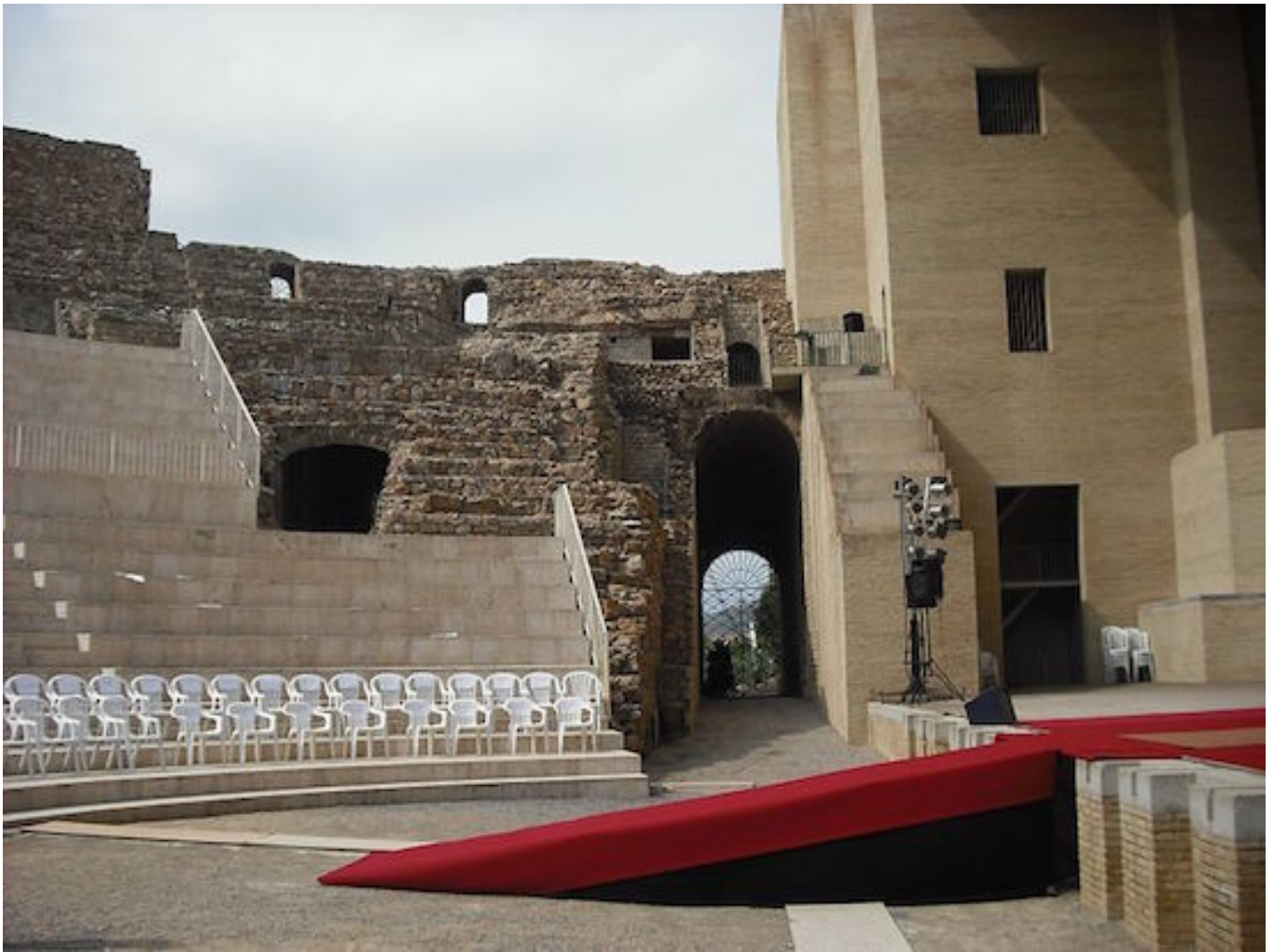
Supplemental brick sceneae frons and Tudela stone cavea seating frame the original stones of the Roman theater in Sagunto, Spain. The design by Giorgio Grassi and Manuel Portaceli was completed in 1993 and received with much criticism. Photo: Iniguez Rodriguez Enrique, Wikimedia Commons.
