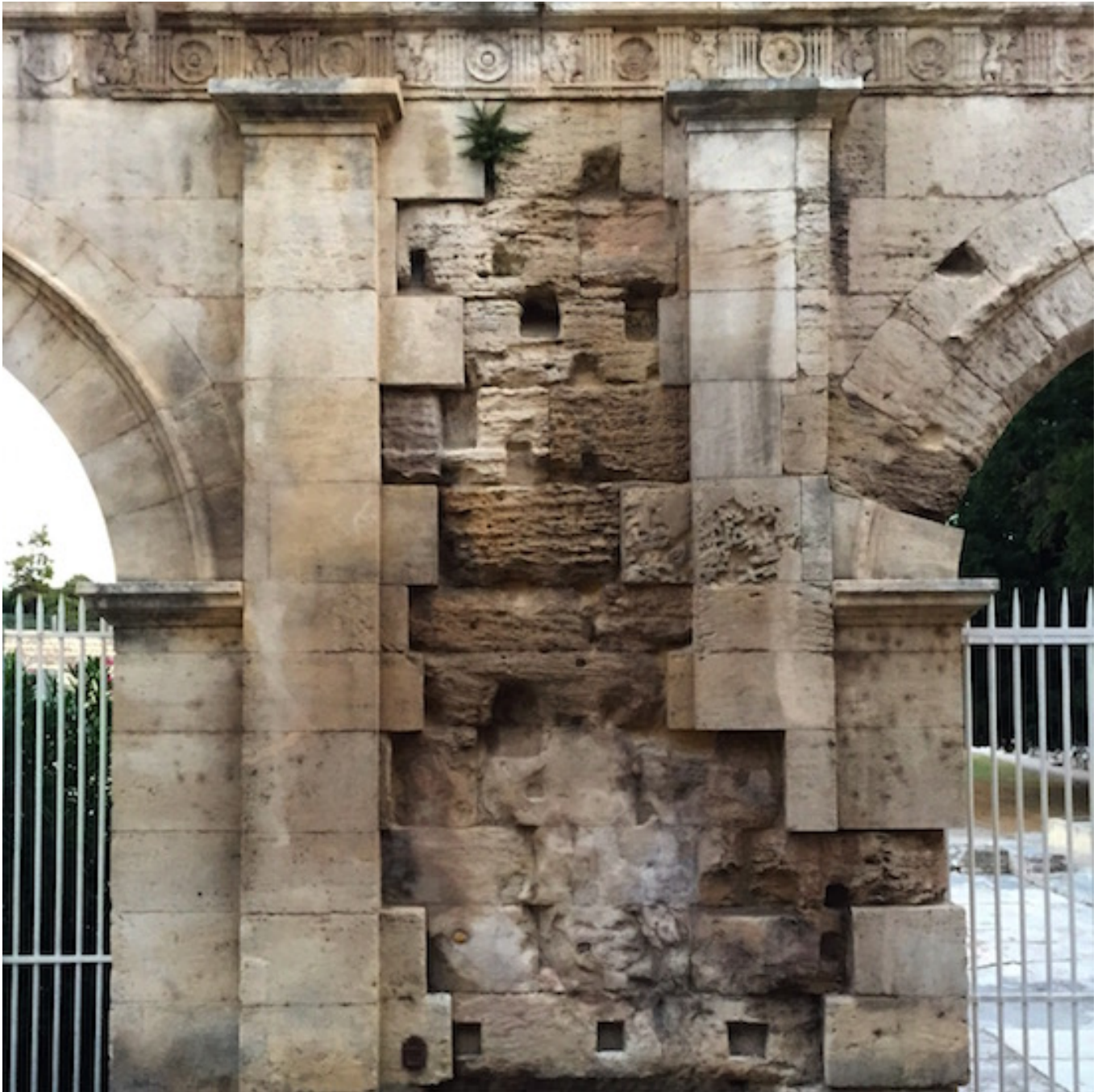
Limestone supplements frame the original stones of the ancient Roman theater in Arles, France. Photo: Jorge Otero-Pailos.
