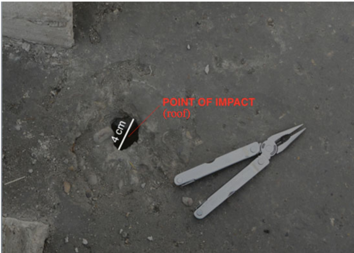
Above: Kent Klich, Tuffah, Northern Gaza, 2009. Below: A much smaller hole was recorded by Chris Cobb Smith, Gaza, 2009. Here the hole is made by a hollow charge – a stream of melted steel. Analysis by Forensic Architecture.
