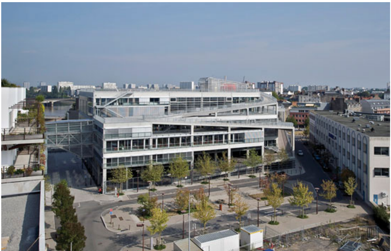
A view of the Nantes School of Architecture, from the Île de Nantes.
