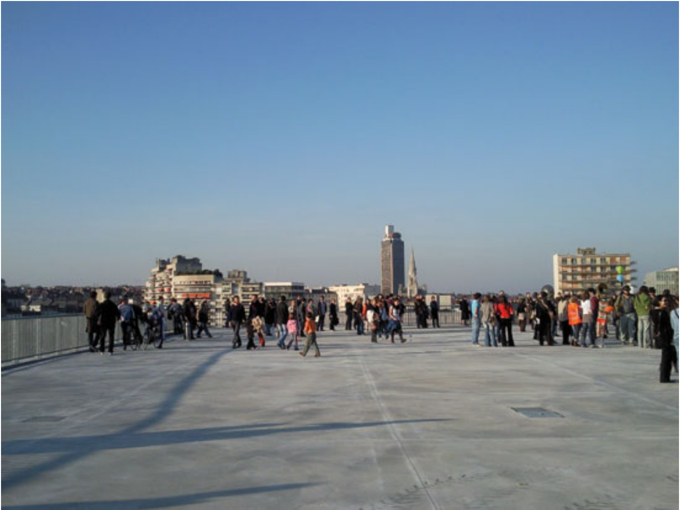
The roof of the Nantes School recalls Bauhaus in Dessau. © Lacaton & Vassal. Photo: Philippe Ruault.
