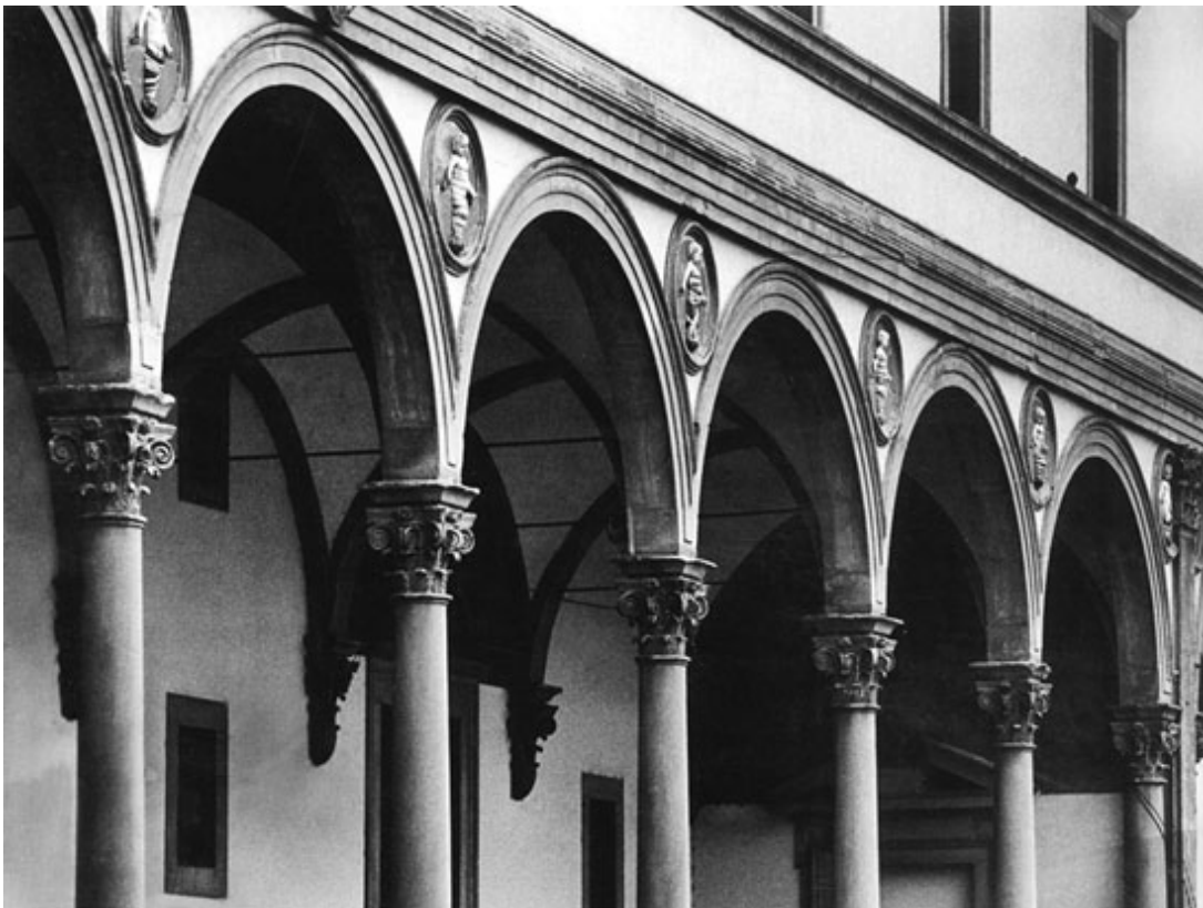
A detail of Brunelleschi's Portico of the Ospedale degli Innocenti exemplifies his use of repeated modules.
