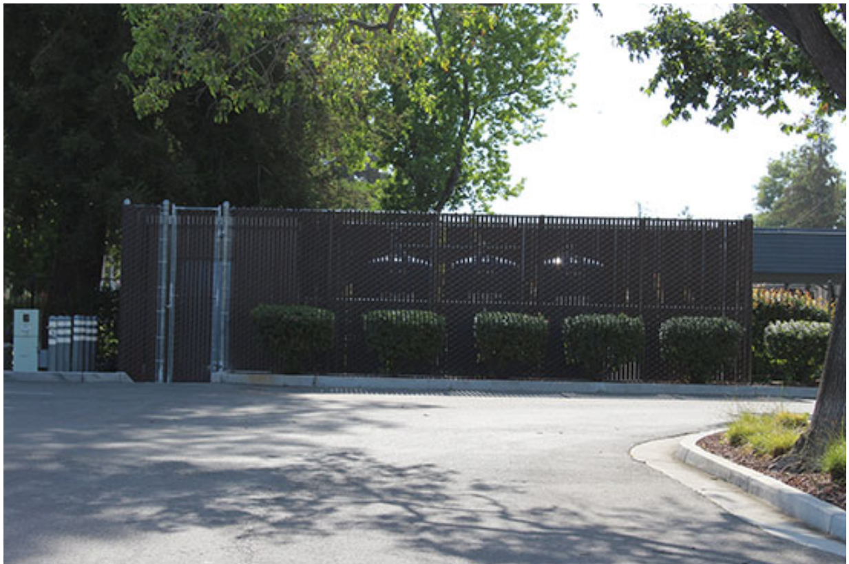
Groundwater treatment pump system at Siemens-Intersil site, Cupertino.
