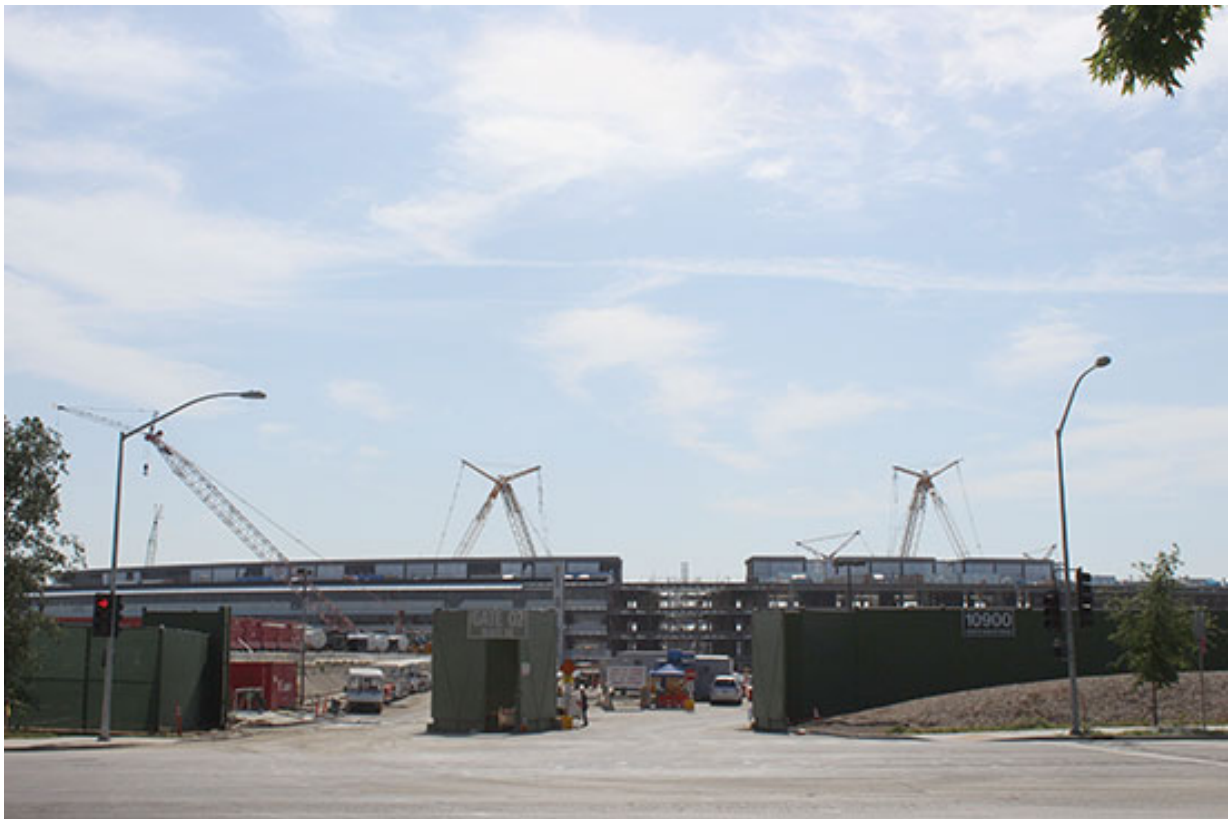
Construction on Apple Campus II, Cupertino. Photo courtesy of the author.
