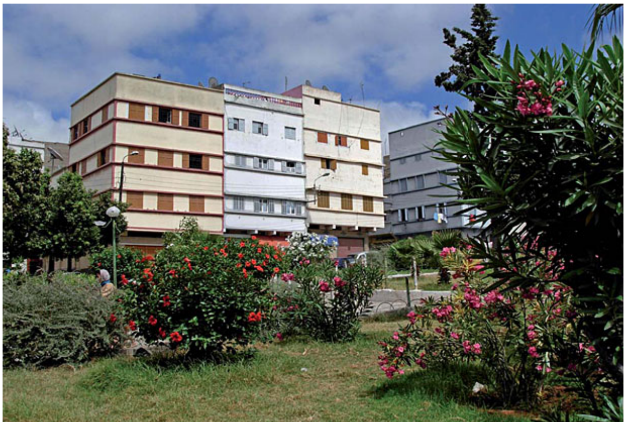
The appropriated Ecochard grid, in which the base structure is used for creating additional apartments on the top of the building. Almost no original structures can be found anymore in the whole town, as all have since been adapted. Casablanca, 2007. Photo: Marion von Osten.
