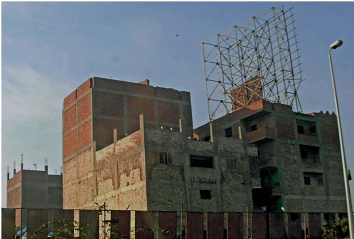
Self-built neighborhood in Cairo, 2009. A simple steel and concrete pillar grid structure reminiscent of Le Corbusier's Maison Dom-ino model. Filled with brick stones, a growing house structure becomes adaptable to the needs and finances of its inhabitants. Cairo, 2009. Photo: Marion von Osten.
