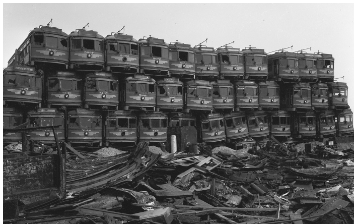
Former Pacific Electric Railway streetcars stacked at a junkyard awaiting destruction in the US, March 1956. License: public domain.
