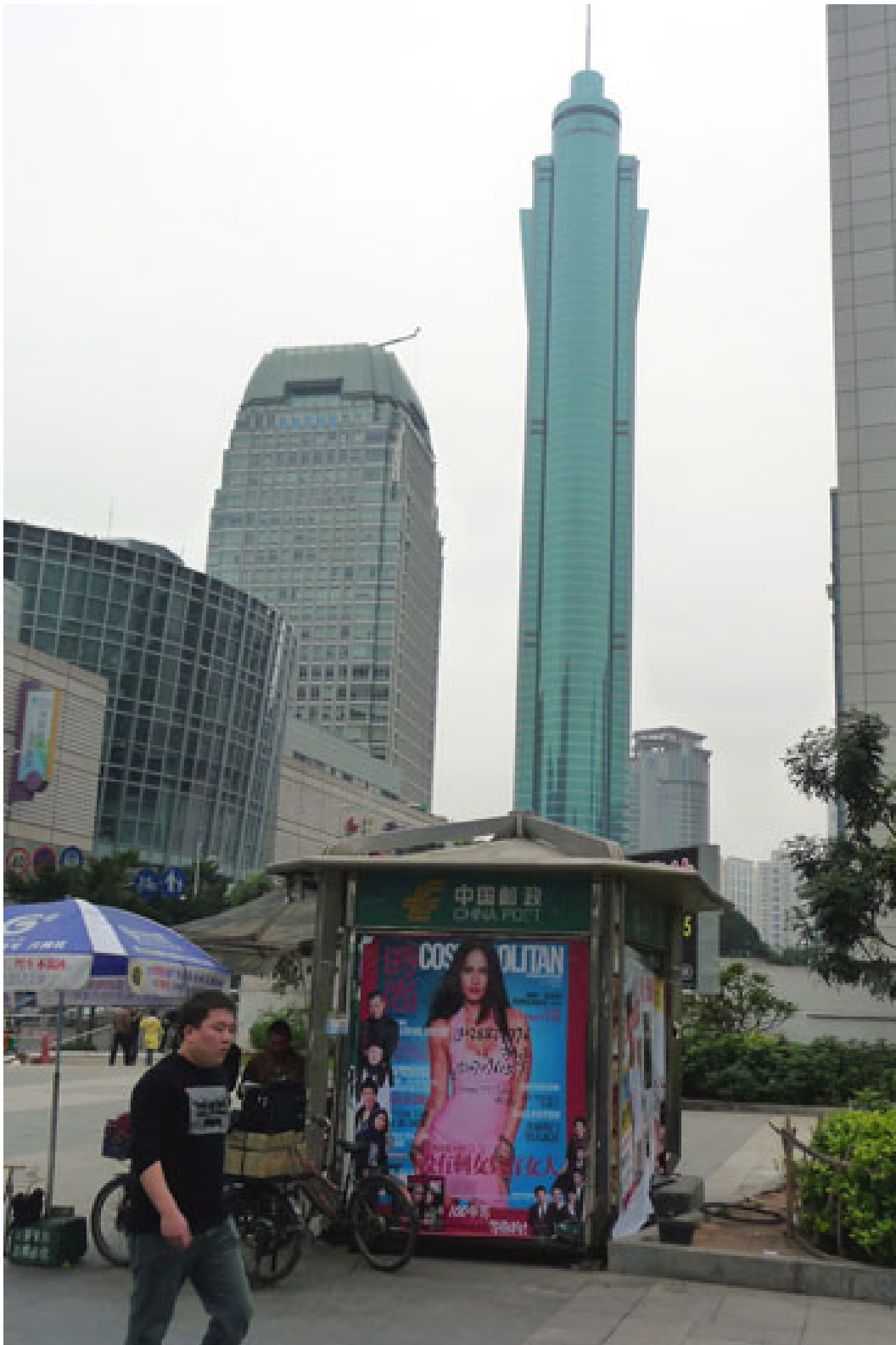
Shun Hing Square tower by K.Y. Cheung Design Associates, Shenzhen, 1996. Already completed in the nineties, the Shun Hing Square tower is one of the tallest buildings in the world that was built at an astonishing speed of four floors in nine days.
